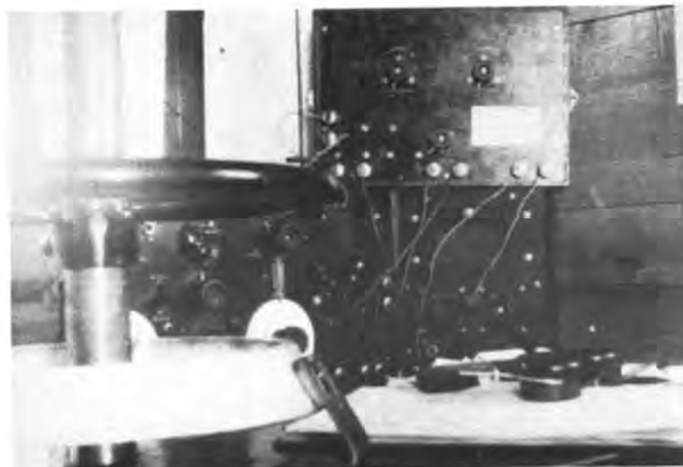
NBD RADIO COMPASS operating position. NOTE "new" R.F. amplifier which has just been "hay-wired" in, according to Carl - also pair of "Baldies" on the desk ! [ Photo - Carl Herr ]
